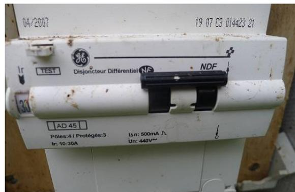
Then swing the bottom of casing out to reveal the switchbox - there's no need to remove the cover entirely - and flip the black switch UP as shown.
